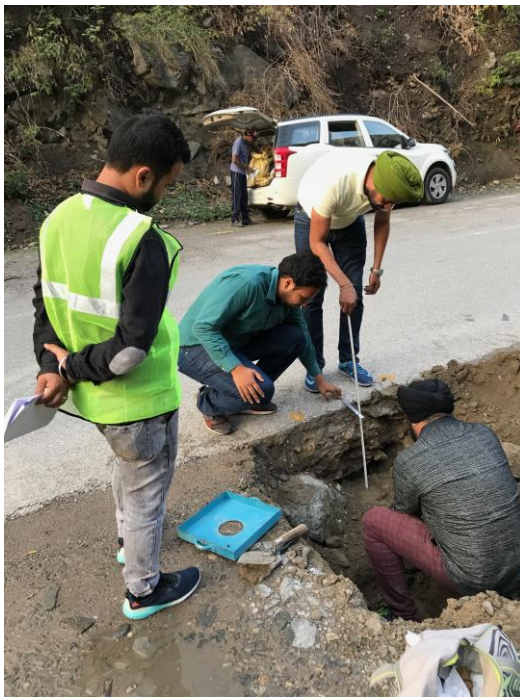
IDENTIFICATION OF PAVEMENT LAYERS
