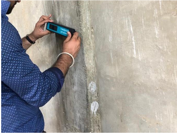
CONCRETE RESISTIVITY TEST
