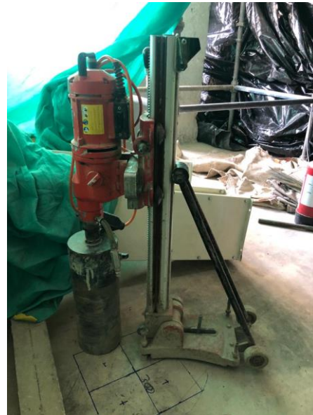
CONCRETE CORE CUTTING
